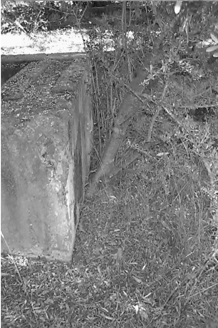
Figure 3.4. Infestation of feral olives between foundations of buttresses.
